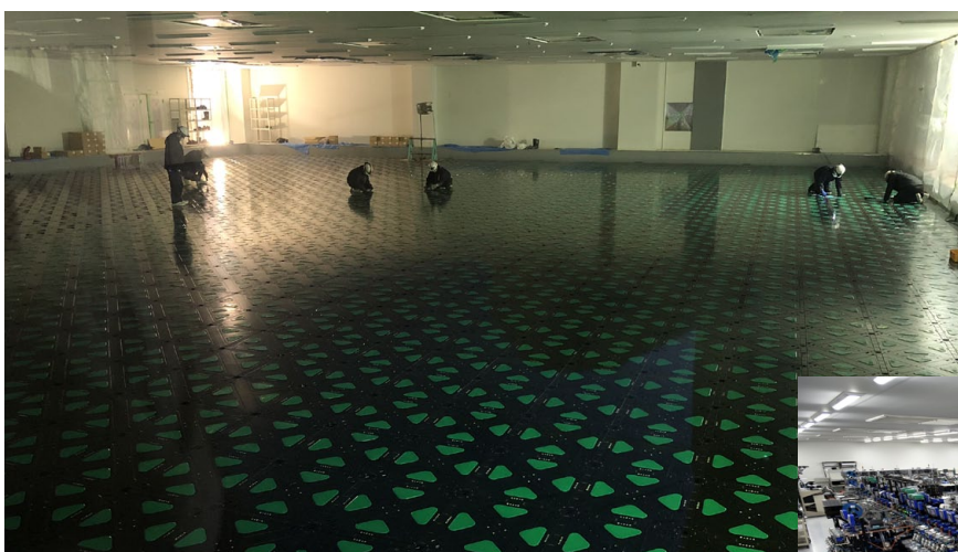
Seismic isolation system for the timepiece manufacturing floor at a new building of Yamagata Casio plant
