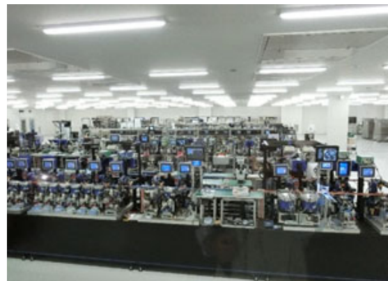
Clean room with latest air-conditioning system
